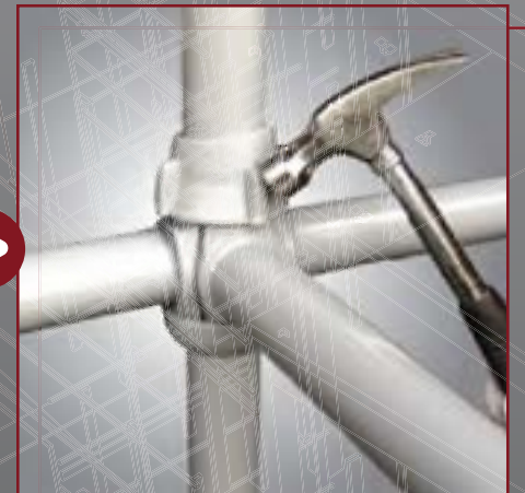
3. Tighten with hammer blow.
